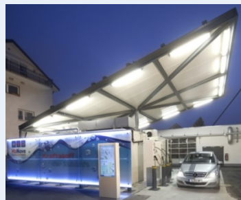
Solar H 2 Filling Station at Fraunhofer ISE
